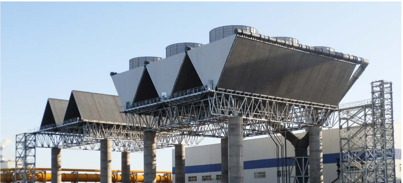
InAIR under construction in China utilizing optional concrete substructure.
