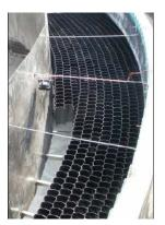
2H TUBEdek® lamella clarifiers can be installed tangentially in a ring at the outer rim of the tank. For this configuration, the width of the ring may not exceed 3 m and the inner diameter of the tank has to be larger than 12 m.
