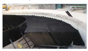
For higher sludge loads and smaller inner diameters we recommend installing the 2H TUBEdek® modules radially. This can be done by cutting the modules into segments like pieces of a cake. The form of the edge profiles allows for an installation without dead ends.
