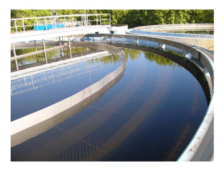
ENEXIO Water Technologies' concepts combine the advantages of the parallel plate separator technology with those of round sedimentation tanks.
