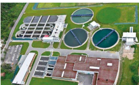
Plant for biological waste water treatment
