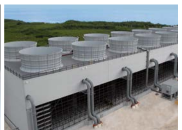
Cooling tower installations
