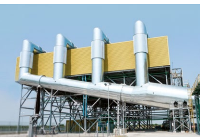
AIR COOLED CONDENSERS
