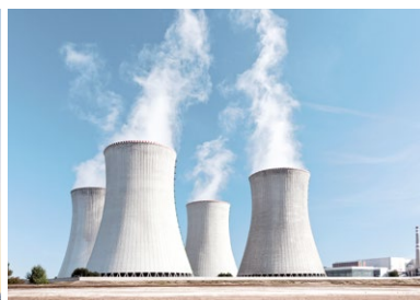
WET COOLING TOWERS
